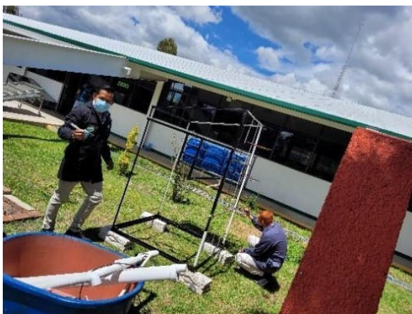
FIGURE 11: Assembly of the structure. Source: Own, year 2022.
